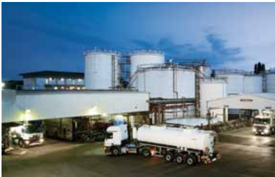
Herne treatment plant: the Herne treatment plant primarily processes, conditions, neutralises and detoxifies hazardous liquids and pasty substances. Its barrel and IBC storage facility has the space to hold up to 240 tonnes of material and its tank farm up to 22,000 cubic metres
