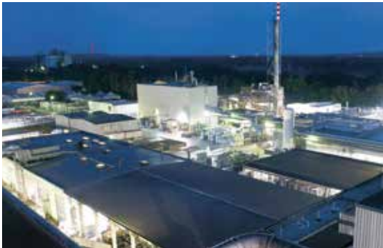
Bramsche Industrial Recycling Centre: over 600 different types of hazardous waste can be safely recycled or disposed of in Bramsche. The high-temperature incineration plant on the site can also treat reactive and toxic chemicals at temperatures of over 1,000°C
