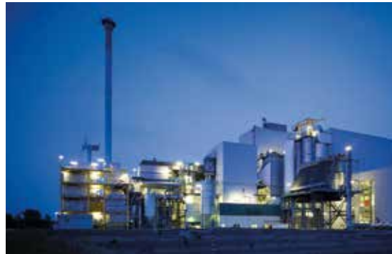
SAVA hazardous waste incineration plant: SAVA in Brunsbüttel specialises in incinerating particularly hazardous waste in a professional and environmentally friendly way. It is considered to be one of the most modern and best performing plants of its kind in Europe for treating solid, pasty and liquid hazardous waste
